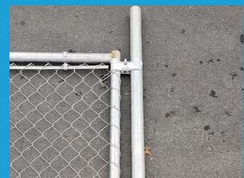
**Step 8- Attach the second post to the other side of the panel with two more clamps.**
